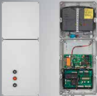
Control unit FS 345 with a backup battery.
